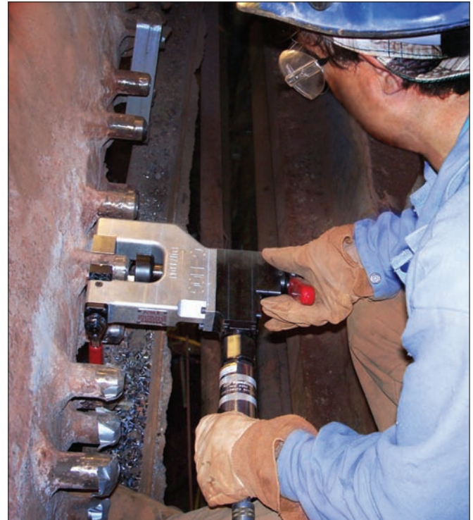
The C-HOG is ideally suited for small bore heavy wall tubes with a high percentage of chrome, stainless steel, and other hard alloys.
